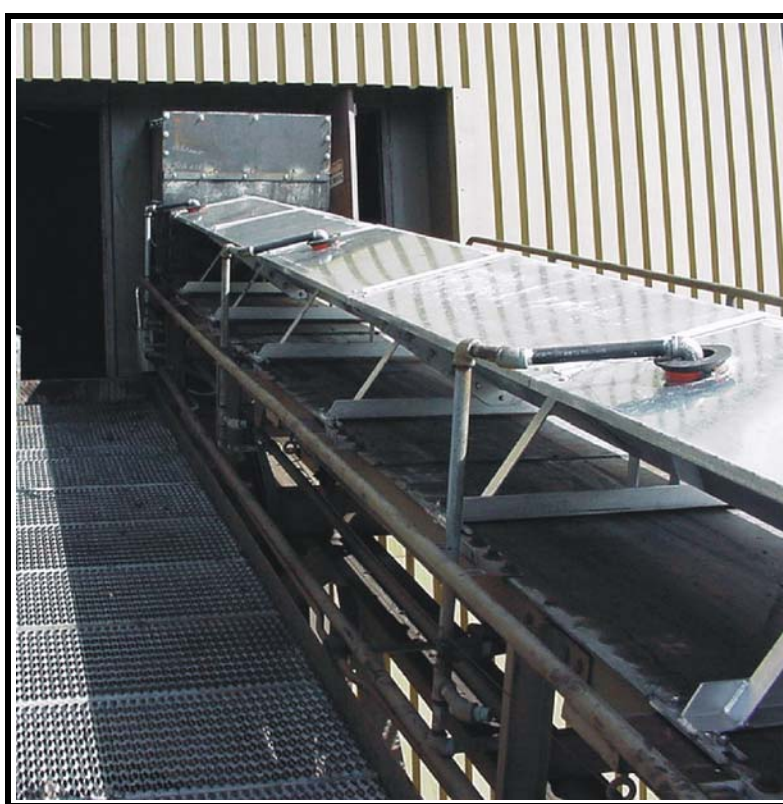
Figure 7. Photos showing installation of a MARTIN® Air-Supported Conveyor
